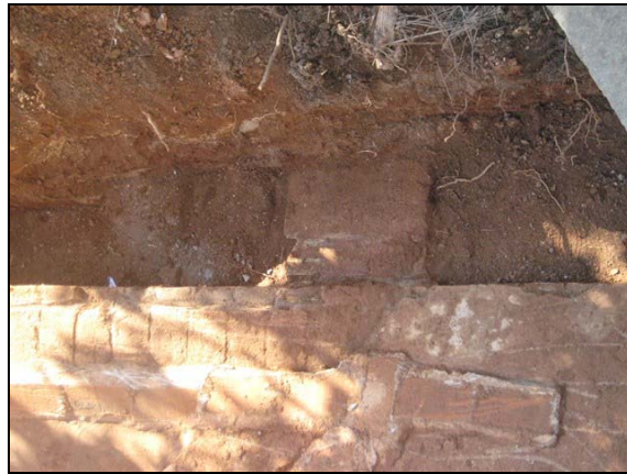
Contrafort de R500b tram 1
